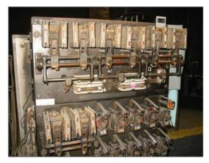
Transite Blocks in Elevator Switchgear
